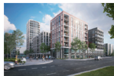
L&Q at Beam Park - Rainham lqhomes.com/beampark
