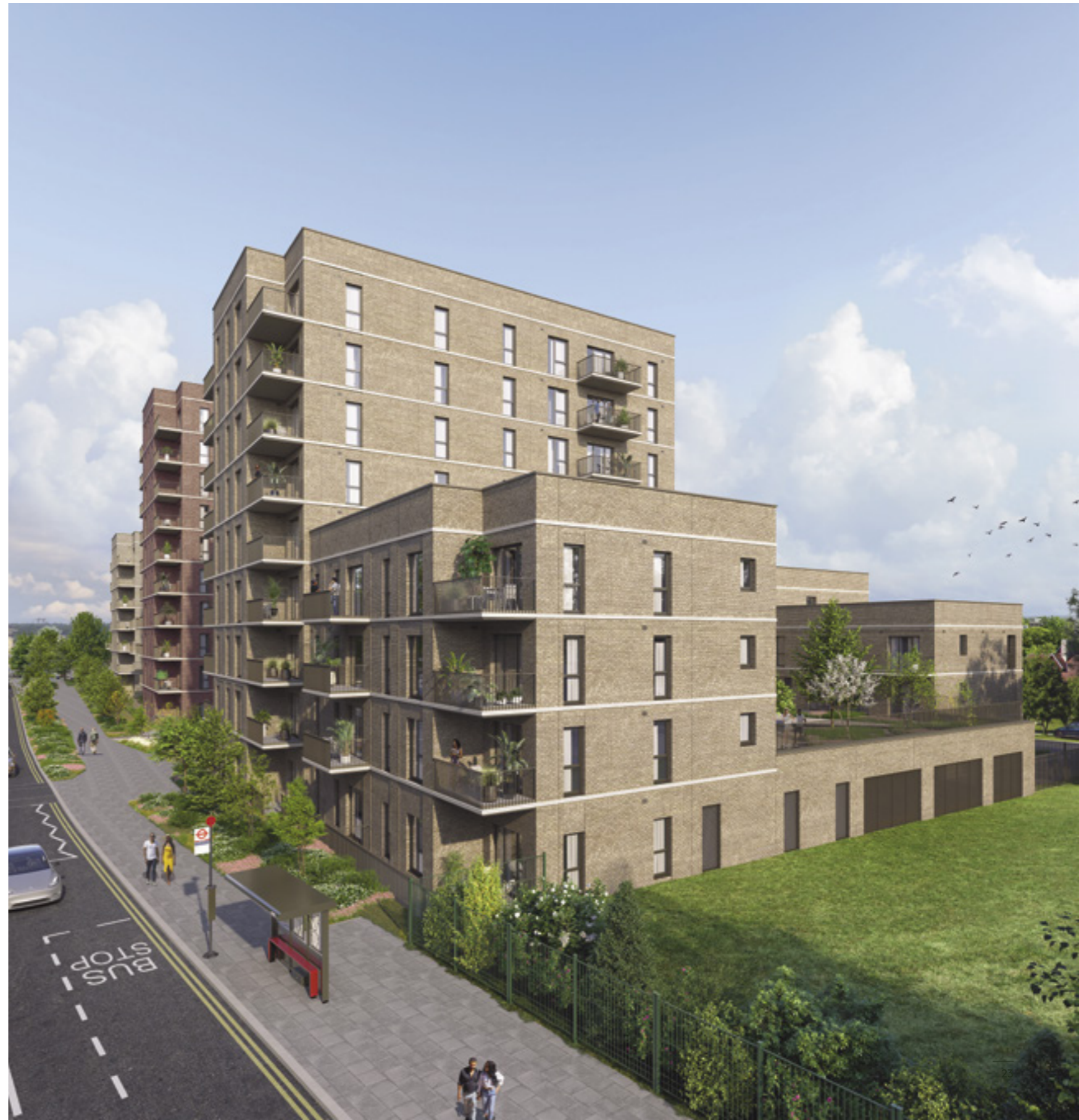
View from New Road south |
