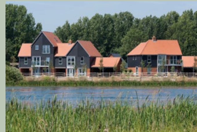
Conningbrook Lakes Ashford, Kent
