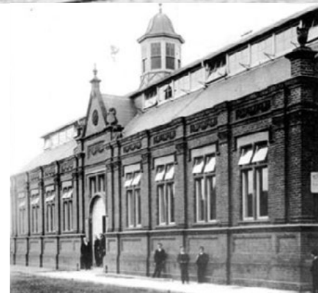
MILL ROAD FREE LIBRARY FRONTAGE (CC.1897)
